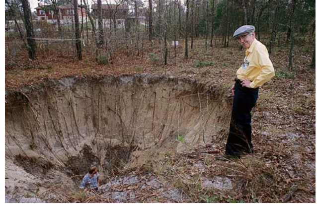
FIGURE 2 A cover-collapse sinkhole that developed rapidly (overnight) near Orlando, Florida. It is approximately 30 feet in diameter and 15 feet deep. Note that only surficial sand (cover) is exposed in the hole. The limestone is approximately 100 feet below the surface in this area. (Photograph courtesy of Barry F. Beck.)
